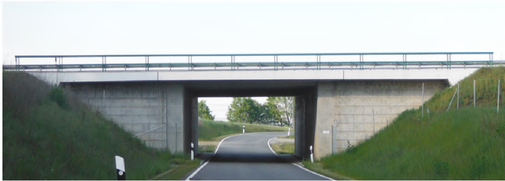
Figure 6. Single-span Concrete Slab Bridge.
